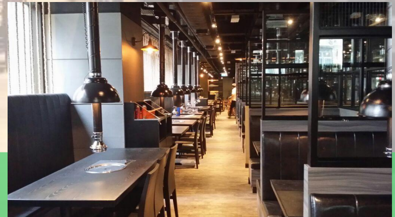
成品 - 冷氣及通風設備 Finished Systems
