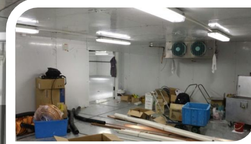
蒸發器安裝 Evaporator installation
