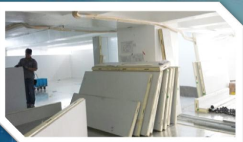
冷庫板預備 Preparation of Cold board
