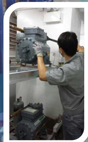
冷庫機組安裝 Units installation
